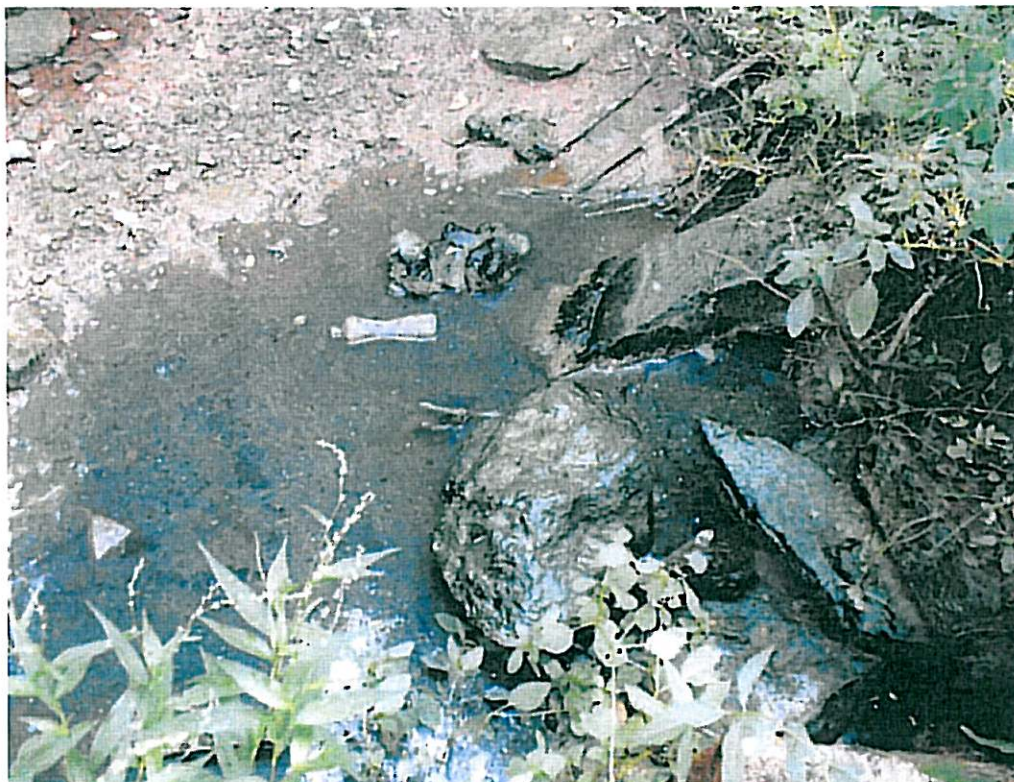
August 14, 2007-Sludge bank at SSO 002.
